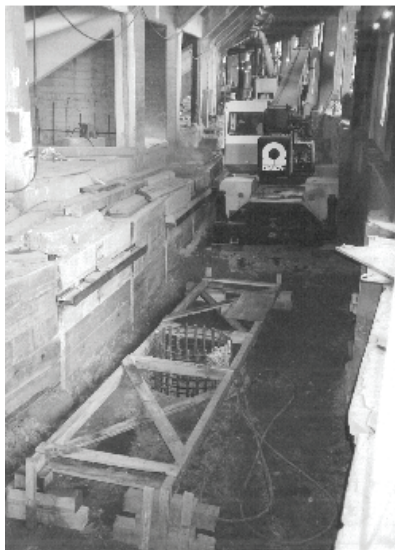
Figure 8 O-cell test under stadium seats
