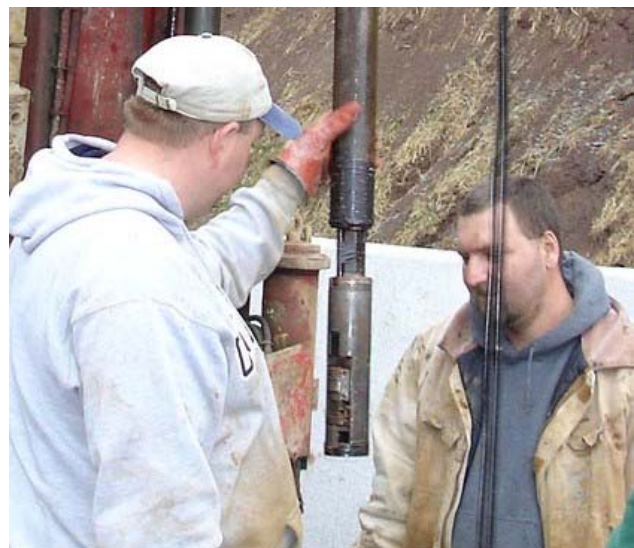
Figure 2: Lowering the rock shear head into the borehole
