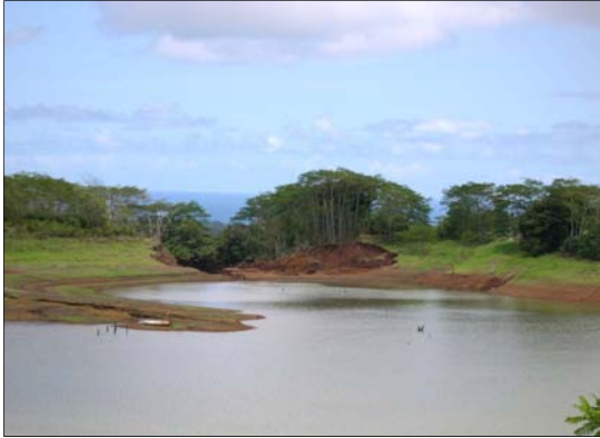
Figure 1 - Breach from rear of the reservoir
