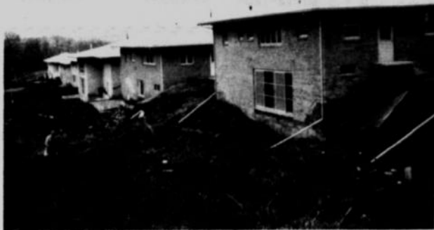
Figure 3. The Aurora Avenue landslide, Des Moines, 1964, and the site of some early Borehole Shear Tests.
