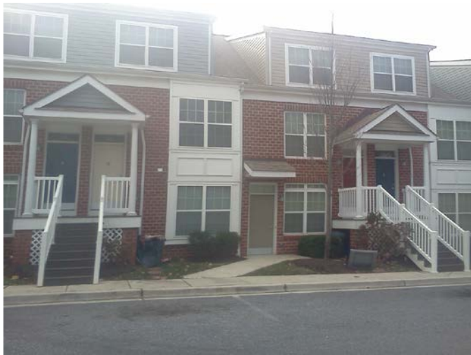
Figure 11: Constructed Buildings for Obery Court
