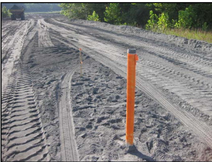
Figure 5B: Completed Settlement Plate--Long term Monitoring
