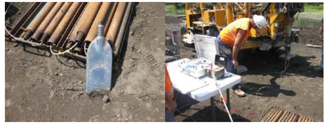
Figure 3: Photos of field testing at site
