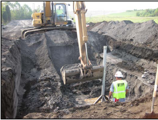
Figure 5A: Settlement Plate Installation
