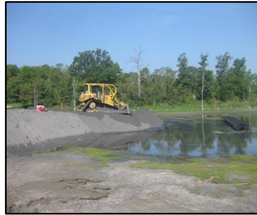
Figure 2F: Access Road Construction
