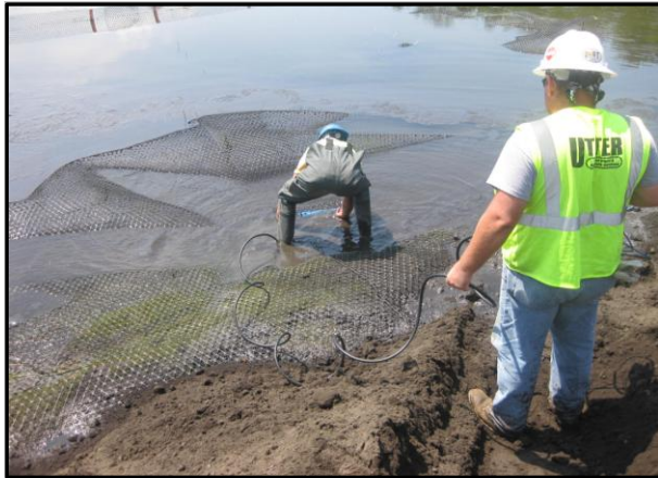
Figure 2E: Porewater Pressure Device Installation
