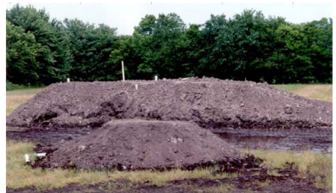
Figure 6: Embankment load test setup
