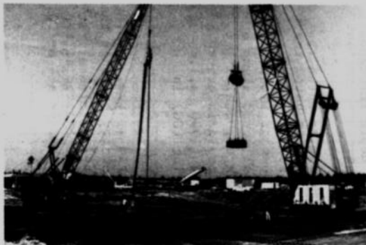
(a) DYNAMIC COMPACTION WORK IN PROGRESS
