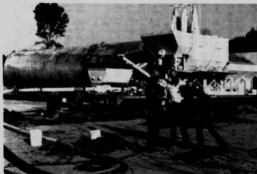
(b) CG EQUIPMENT IN OPERATION
