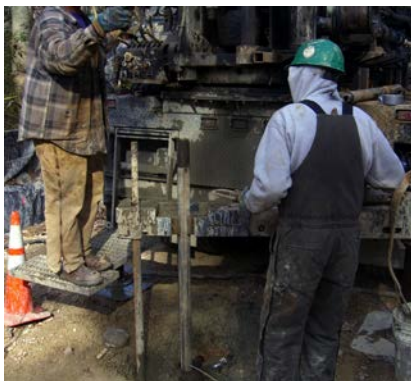
Figure 9: Break-out Wrench/Rod Clamp
